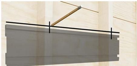
Using your preferred method, locate and mark every stud along the line. Transfer stud marks into top and bottom channels.
